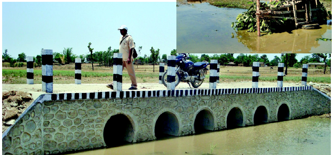
Community culvert bridge before & after
