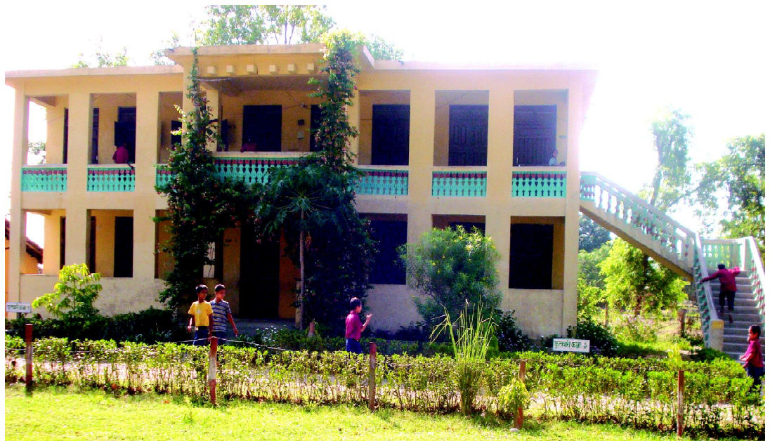
Building of model school of Kailali district
