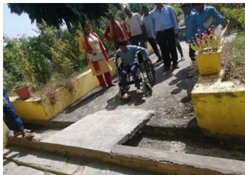
Corridor entrance without ramp
